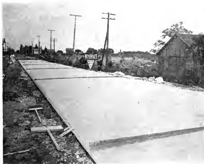
Fig. 1.—Expansion joints are placed every 35 ft.
